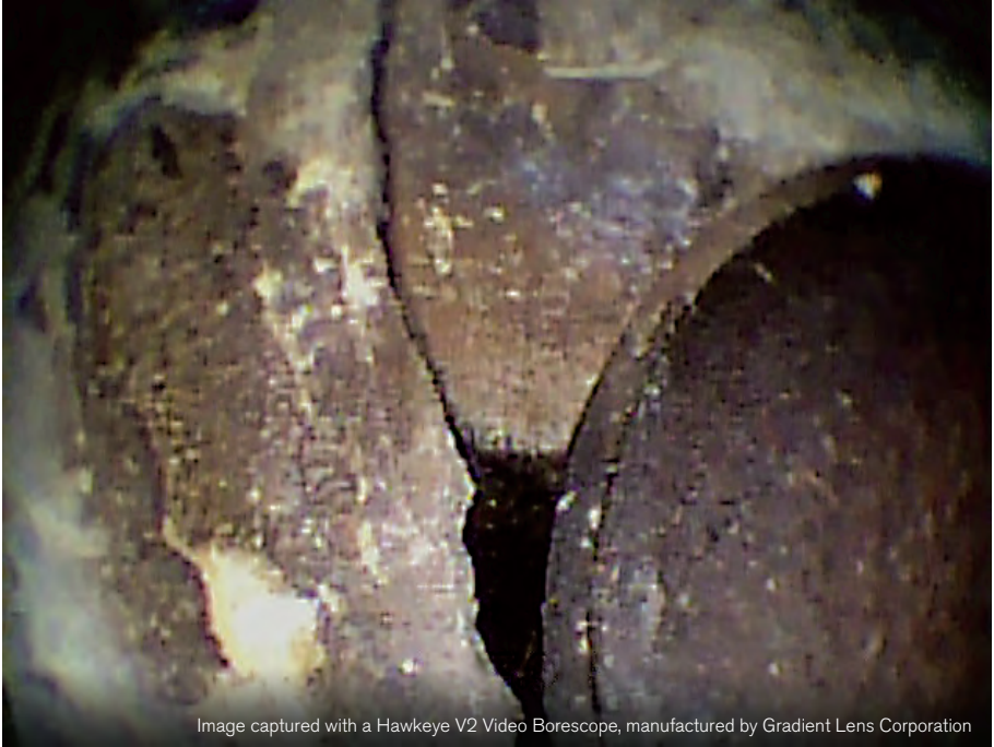
Damaged valve seat as seen through a video borescope.
