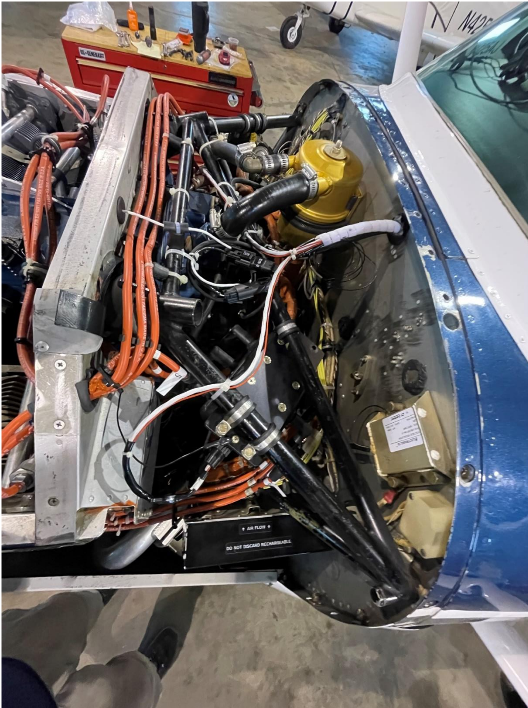
Electroair cable harness routing through the firewall
